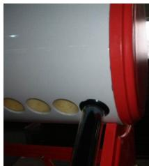
Step 16: Installing vacuum tube one by one
